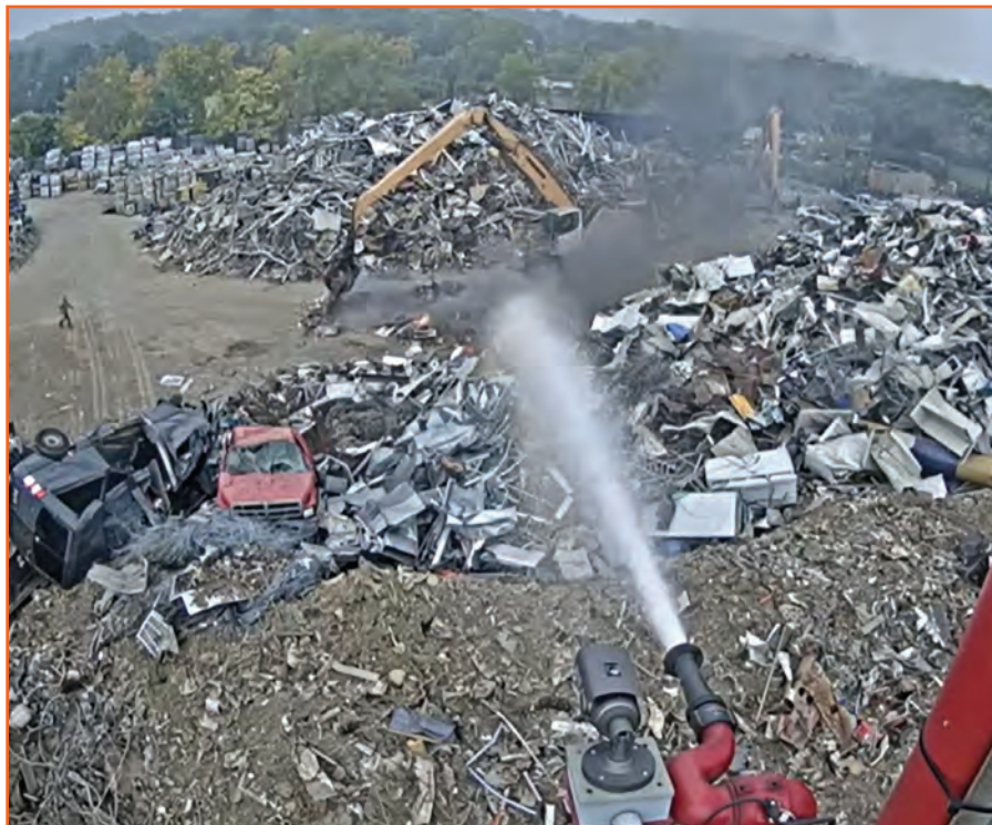
High-tech fire detection and suppression systems—such as this one from Fire Rover—identify hotspots, smoke and fires early, notify local firefighters and then spray an environmentally friendly cooling agent around the problem area to slow down or prevent thermal runaway.
